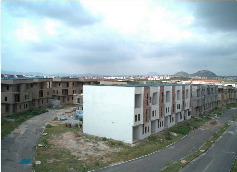
ACTUAL SITE PHOTOGRAPH — Terrace block, end elevation
