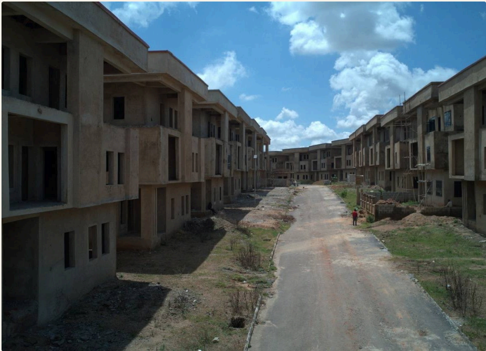
ACTUAL SITE PHOTOGRAPH — Internal estate road
