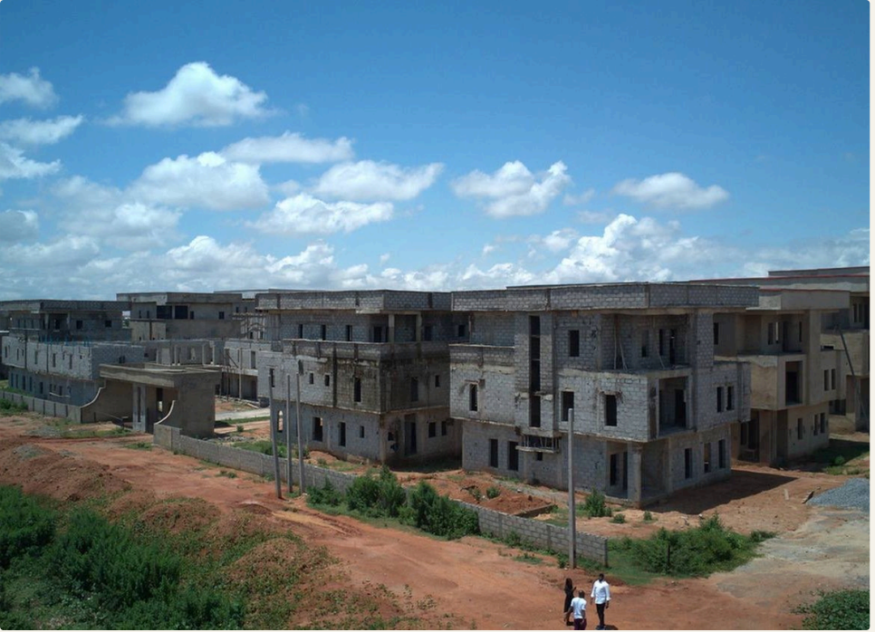
ACTUAL SITE PHOTOGRAPH — Buildings at advanced carcass stage
